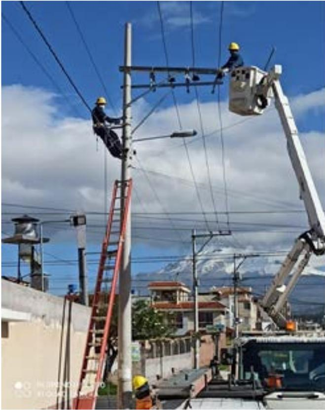
**Figura 2.***Instalación de reconectores*
