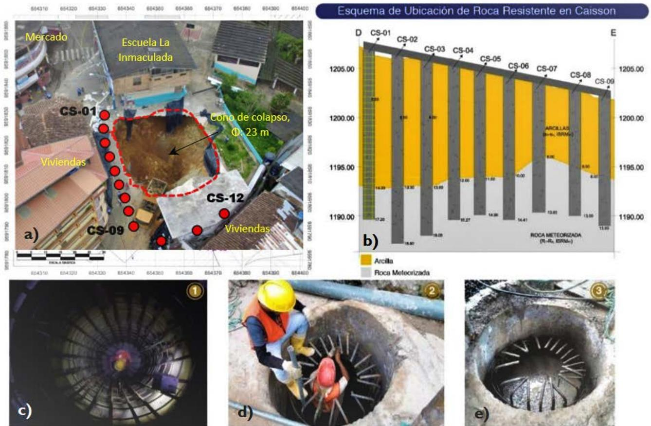
Figure 3. Location (plant and profile) and caisson-type stilt construction process (CS-#)
