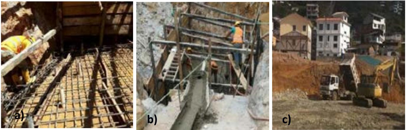
Figure 4. a) mortal level + drains + viga perimetral + armed with iron, b) slab cast, c) fill with class three sub-base compacted material
