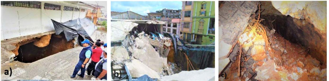
Figure 2. a) collapse start with 10 m cone, b) unstable structures, c) rubble (columns, hoses, cables, blocks) inside the gallery that caused the ground subsidence on the surface
